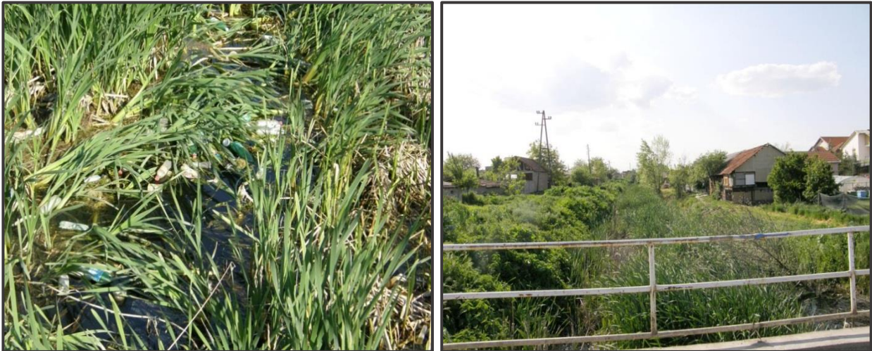
Picture 1: Conditions of the sewage system (in 2015)
