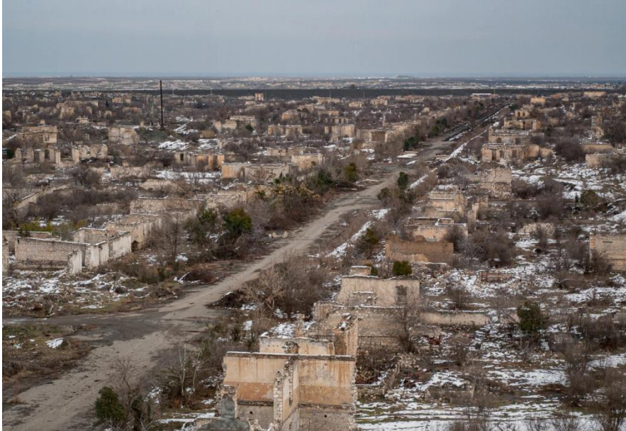
Aghdam City Destroyed by Armenia – Urbicide in Aghdam
