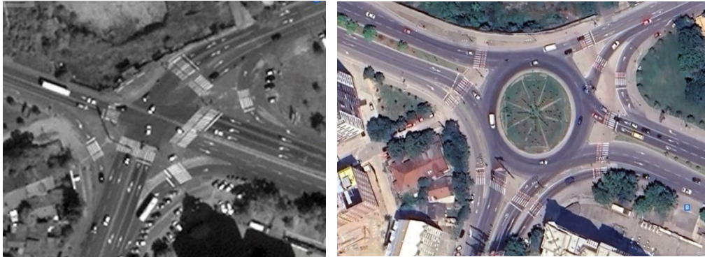
Figure 10. The intersection of the Partizanski odredi boulevard and the Aco Šopov street in Skopje, before and after implementing the flower-shaped roundabout
