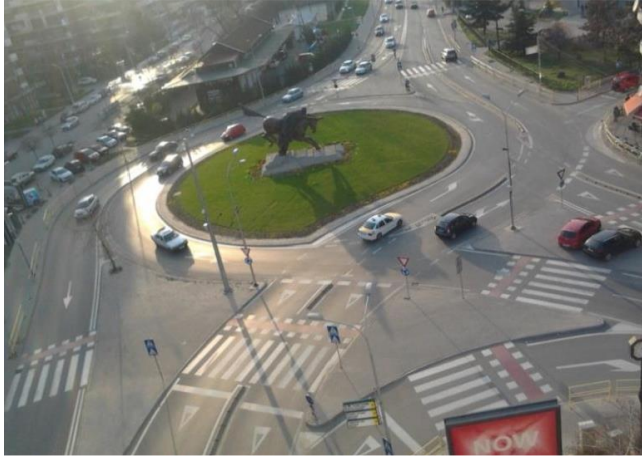
Figure 3. The first turbo-roundabout in N. Macedonia – the M. T. Gologanov street and the Sv. Kiril i Metodij street in Skopje
