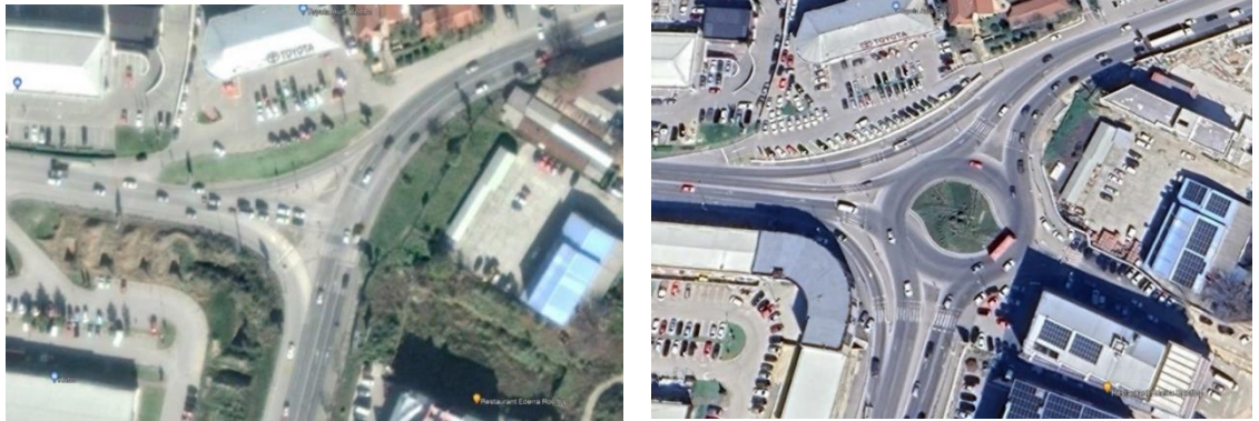
Figure 8. The intersection of the 8. Septemvri boulevard and the Skupi street in Skopje, before and after implementing the turbo-roundabout
