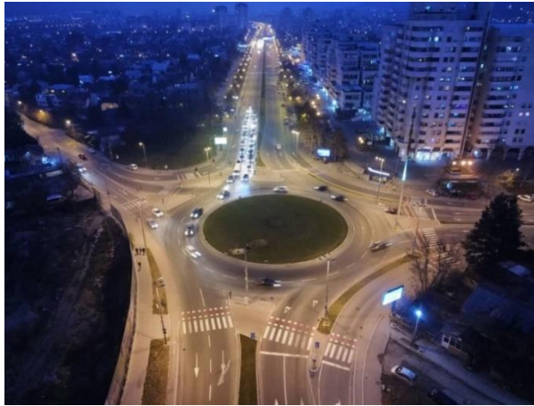
Figure 11. Flower-shaped roundabout at the intersection of the Partizanski odredi boulevard and the Aco Šopov street in Skopje
