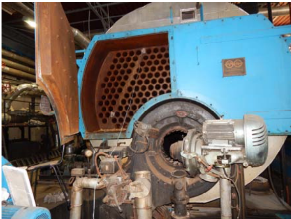
Fig. 1 Installation of temperature probes
