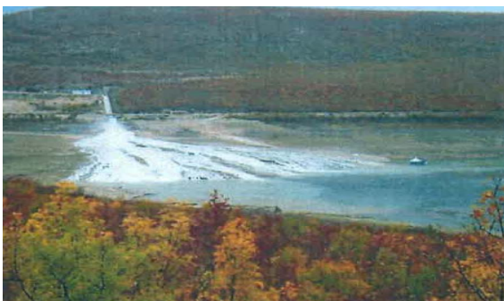
Fig. 12 Location of the powerhouse of HPP Bileća [11]
