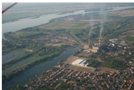
Fig.2. Connection of the Kostolac thermal power plant with the Danube
