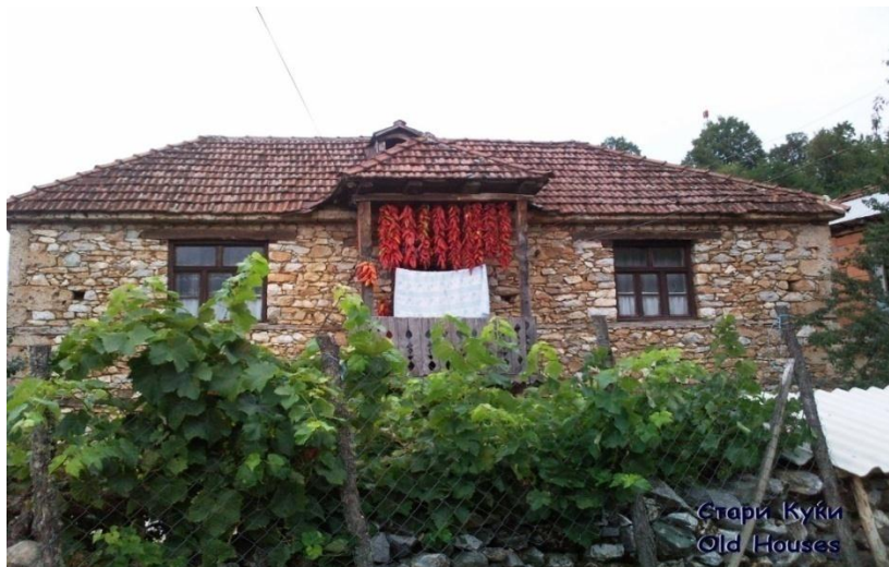
Picture no. 20: Old house in the municipality of Debrca
