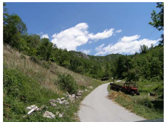
29 View from the existing road passing under the newly viaduct to the church Holy Annunciation
