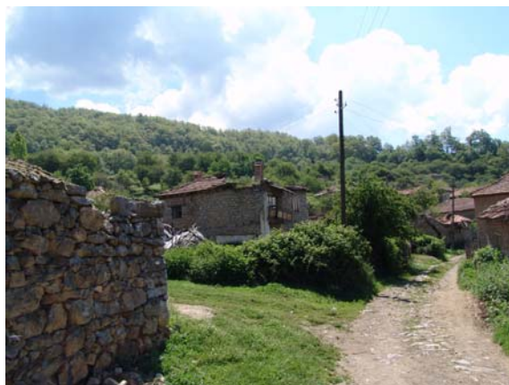
56 Existing road to the Konjsko settlement
